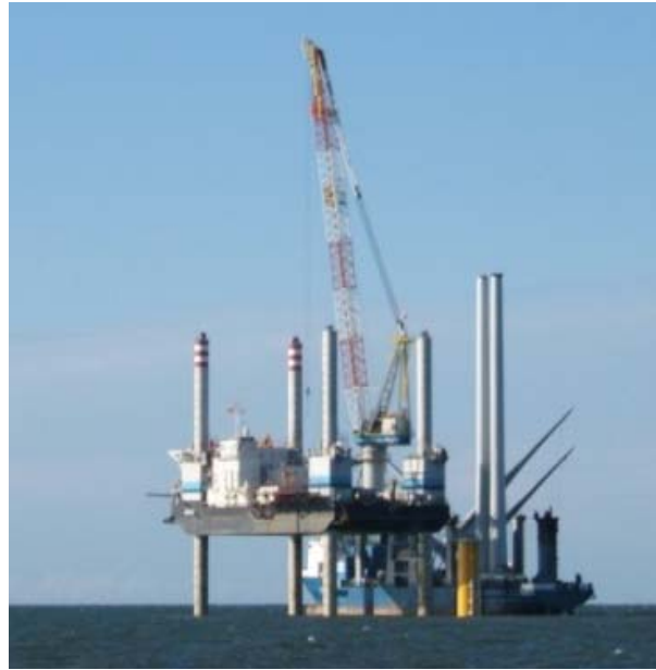
Offshore installation of turbine tower
