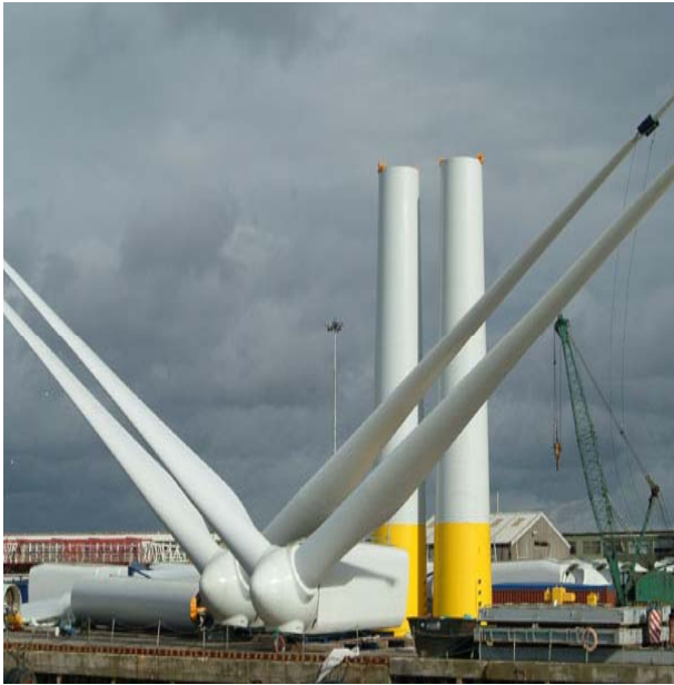
Pre-assembled turbine parts in the harbour
