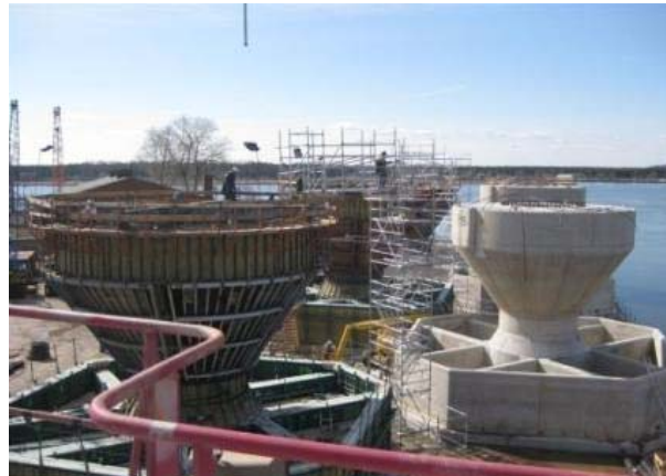
Foundations are cast in concrete
