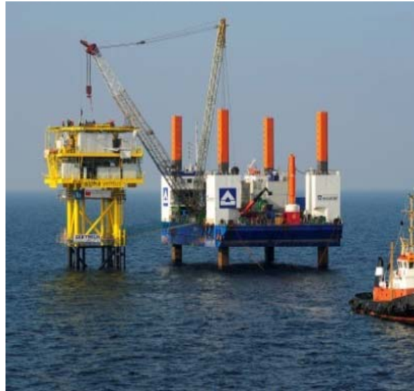
Transformer topside installation
