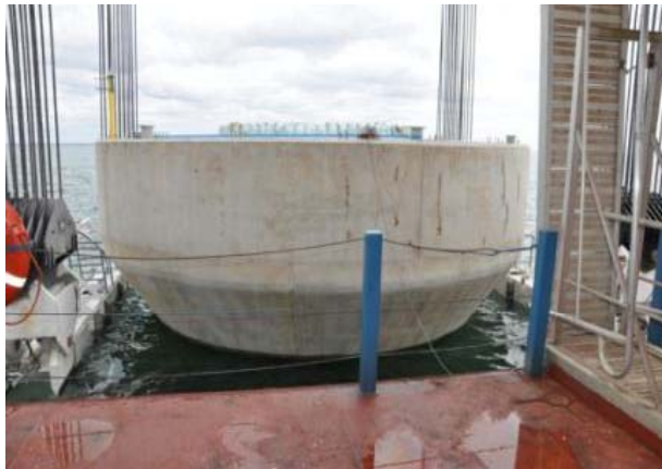
Foundation being lowered to seabed
