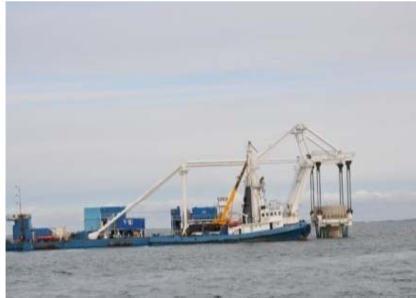
Heavy lift vessel on site
