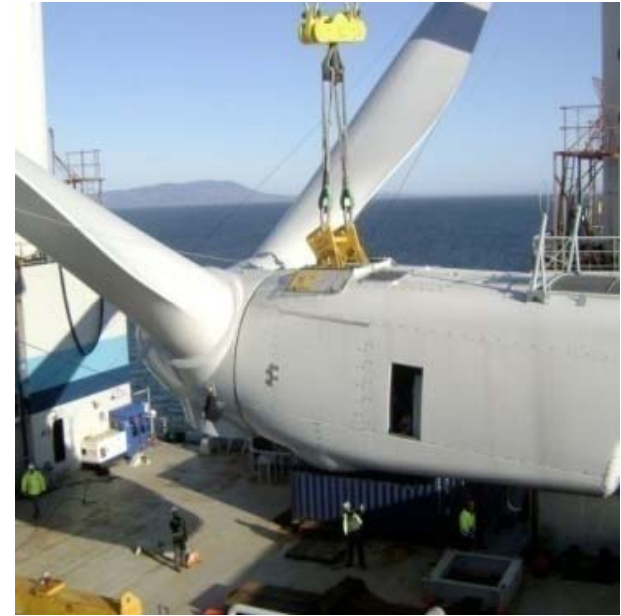
Turbine nacelle being lifted
