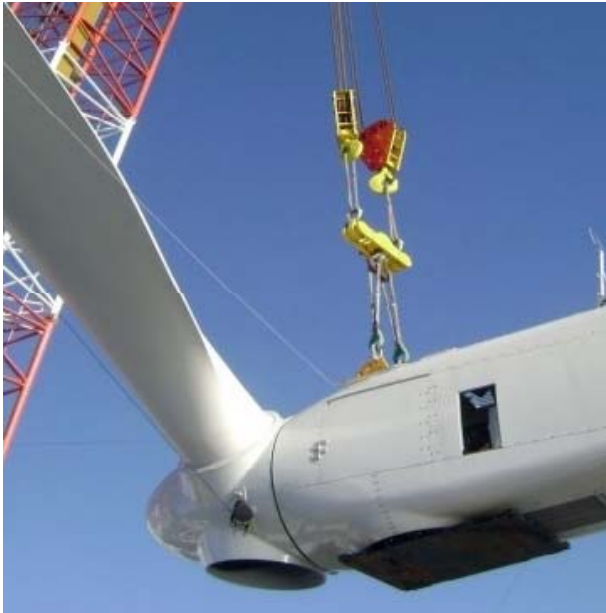
Turbine nacelle being positioned on tower
