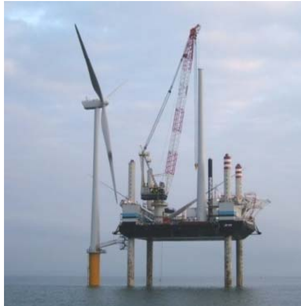
Installation of the third turbine blade
