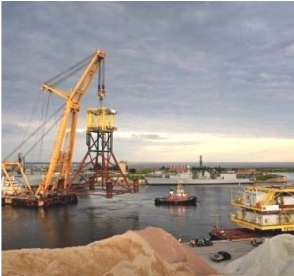
700 ton jacket foundation being transported
