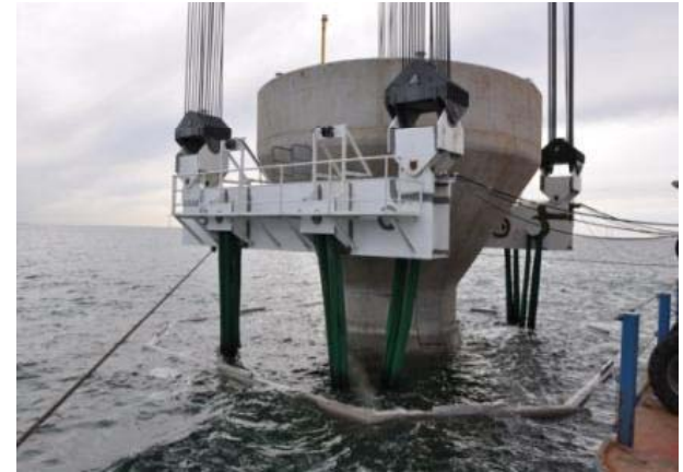
1,300 ton foundation being positioned
