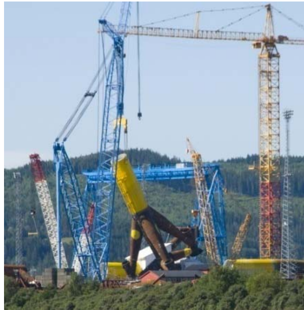
Tripod up-ended for shipping
