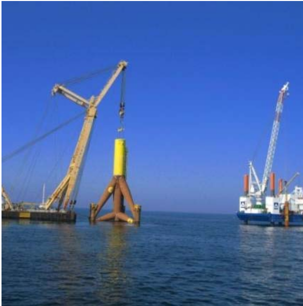
Heavy-lift crane ship on site
