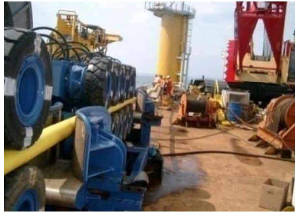
Cable pulling to foundation
