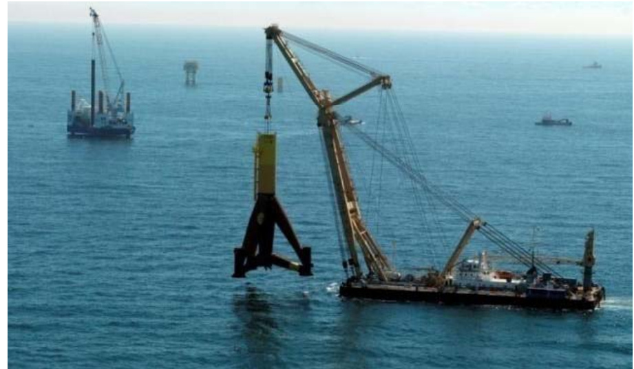
Heavy-lift crane ship during foundation installation
