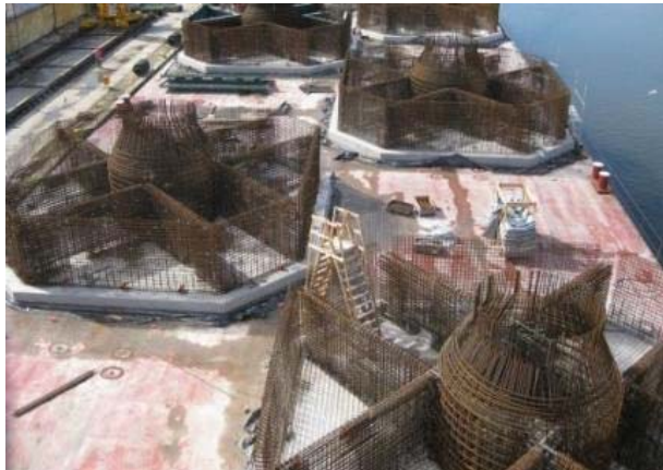
Construction of the steel formwork
