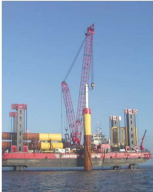
Pile hammer (300t of force) driving monopile
