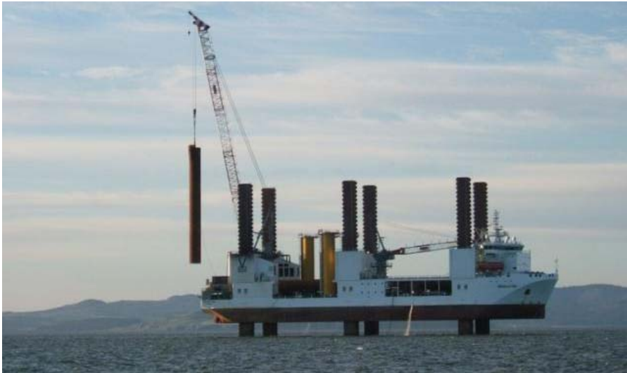
Jack-up crane vessel during foundation installation
