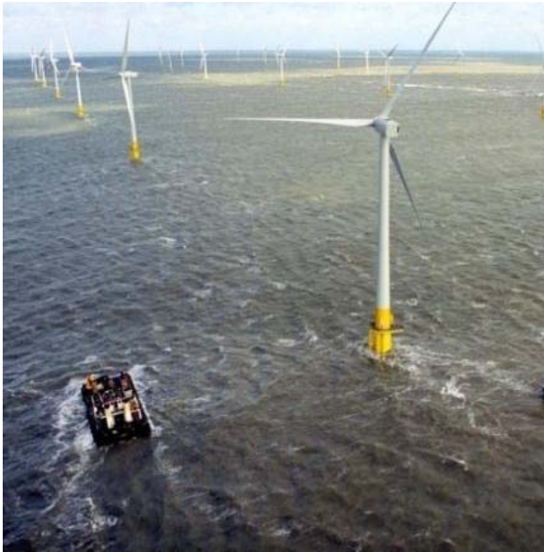
O&M vessel arriving on site
