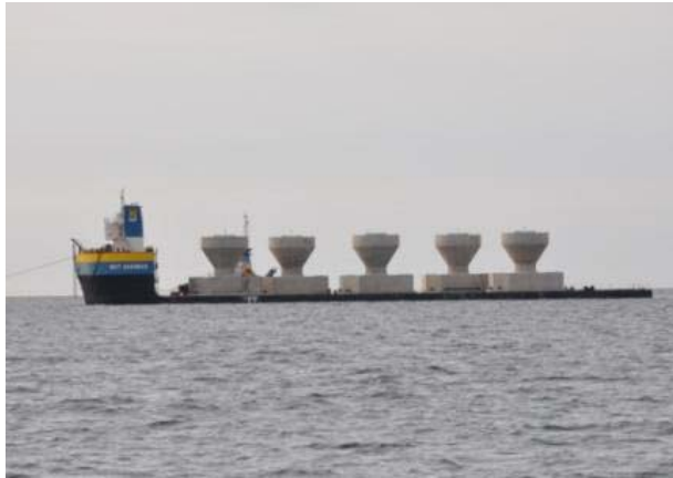
Foundations being shipped to site
