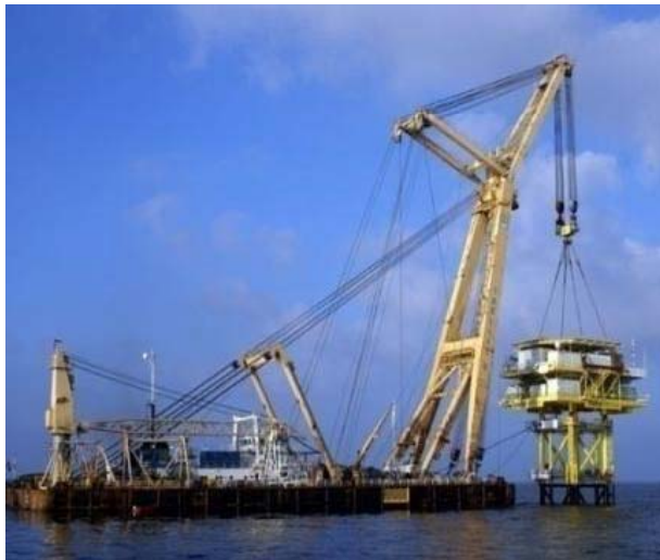
Heavy-lift crane ship
