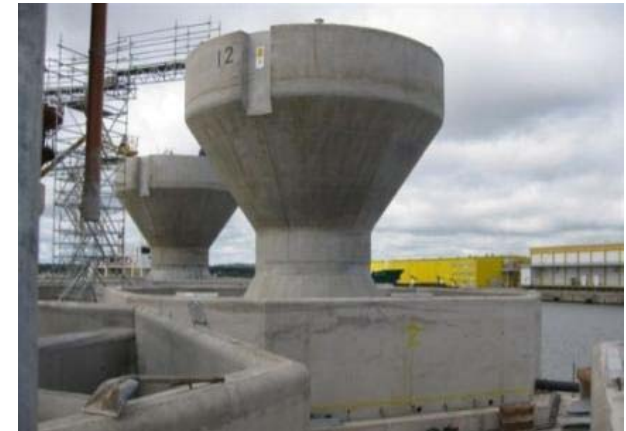
Completed gravity foundation
