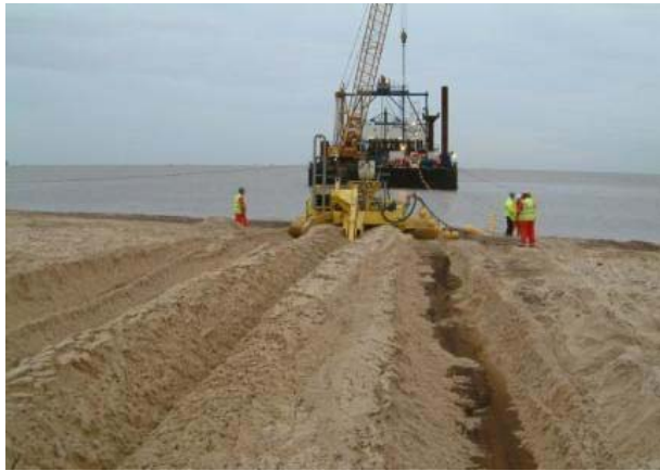
Cable plowing on shore
