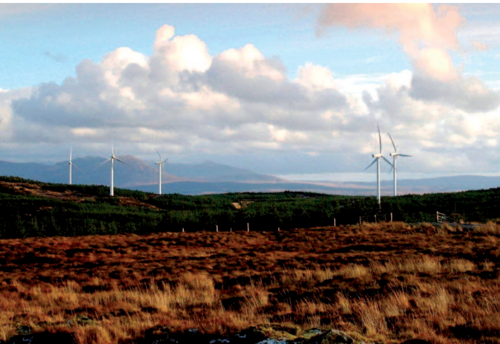
Our Deucheran Hill wind farm, near Carradale, Kintyre.
