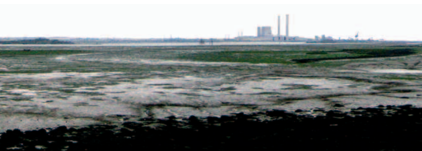
Figure 3c Proposed distance view of units 5 & 6 from Sharp's Green Riverside Country Park and Saxon Shore Way, Rainham, after demolition of the existing units.
