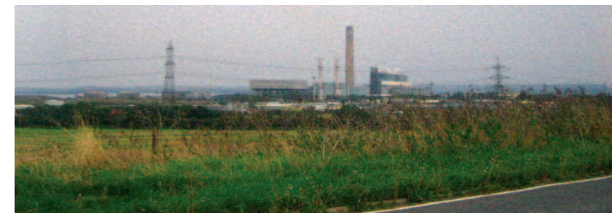
Figure 5a Existing view from Tunbridge Hill, looking towards Kingsnorth Power Station.
