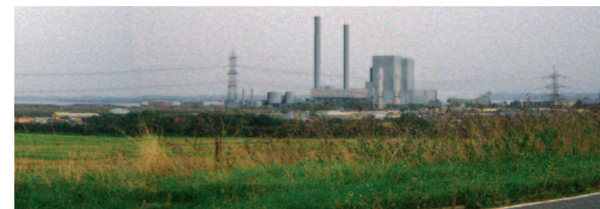
Figure 5c Proposed view from Tunbridge Hill, looking towards Kingsnorth Power Station, after demolition of the existing units.
