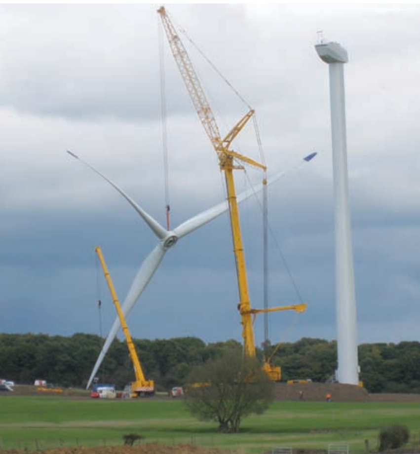
Turbine installation at Butterwick Moor Wind Farm, County Durham
