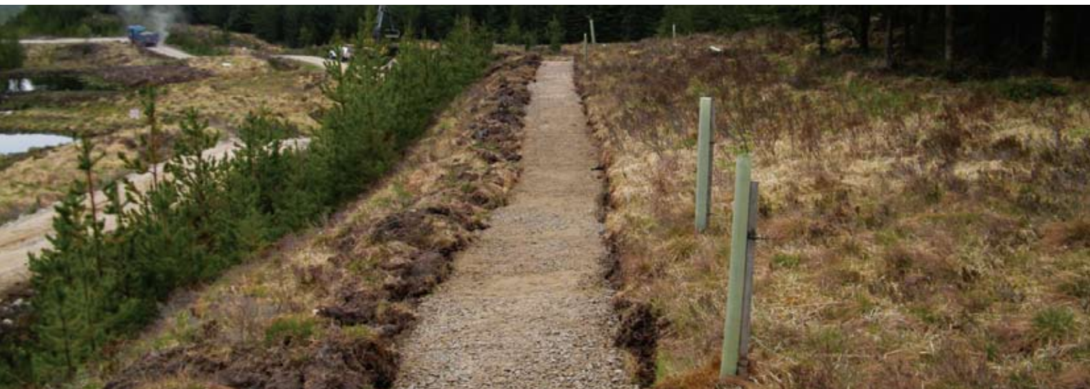
Construction of the Sika trail diversion
