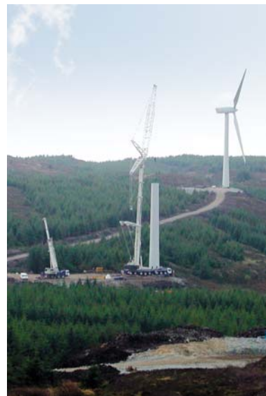
Construction at Deucheran Hill Wind Farm, Kintyre.
