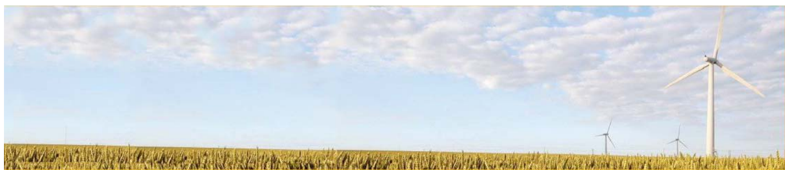
Photo of Out Newton Wind Farm, Yorkshire.
