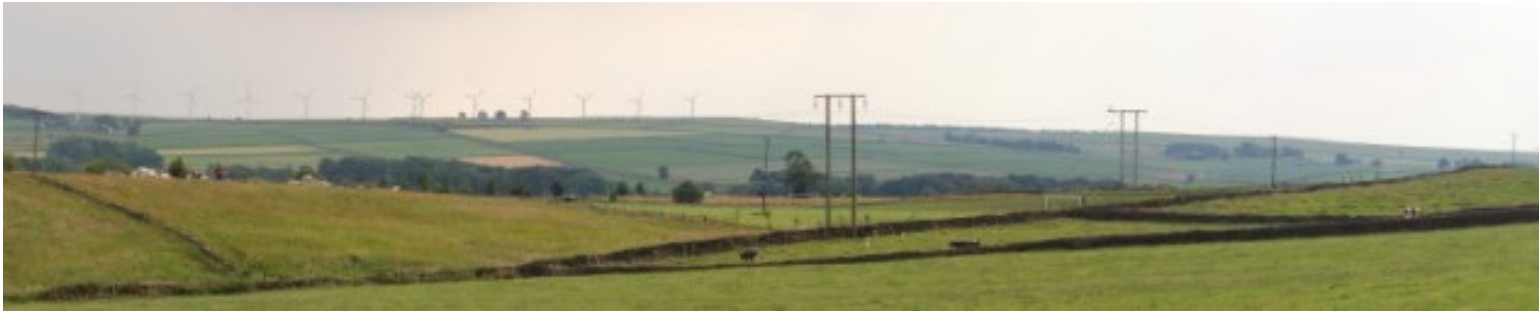
Above shows view of existing Royd Moor farm from A629, High Flatts, Grid Ref: E421848, N406555
